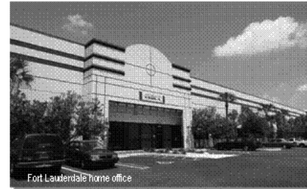
Fort Lauderdale Home office
